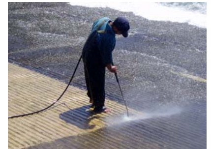
'Bwiden' water blasting slimes.
