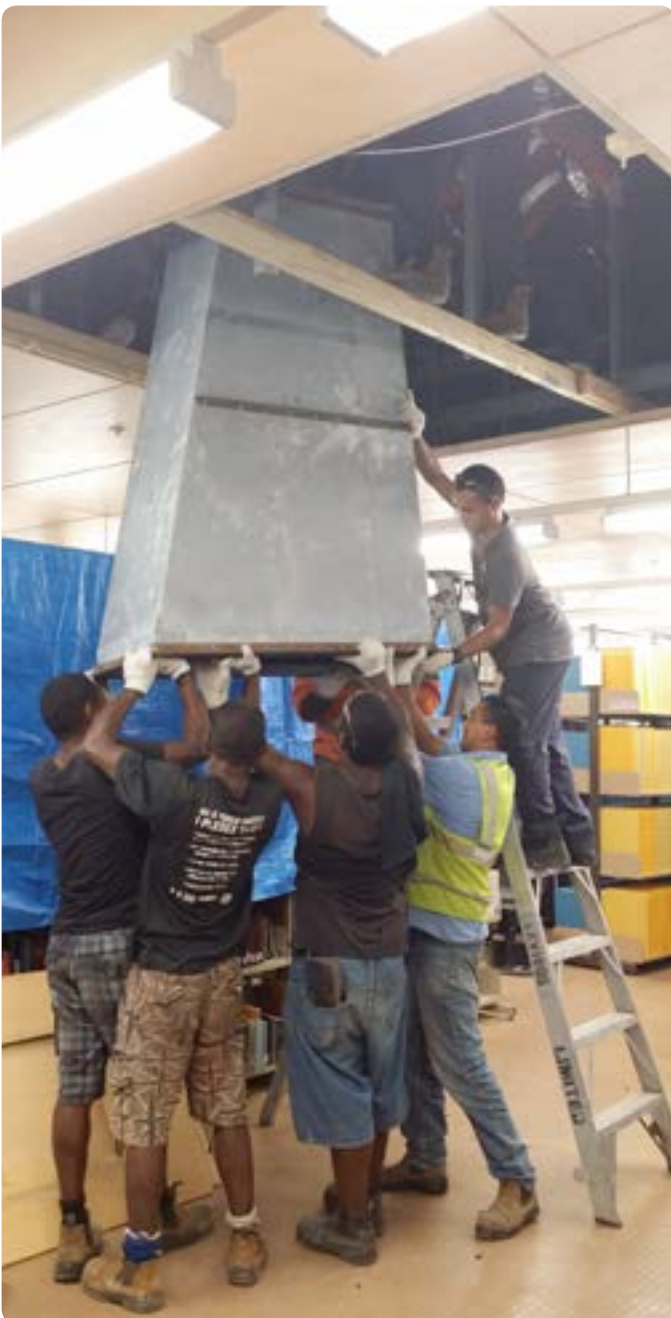
Staff from Mechanical Services removing the old air conditioning ducting.
