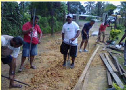
IAS Staff Construct HART Village Footpath
